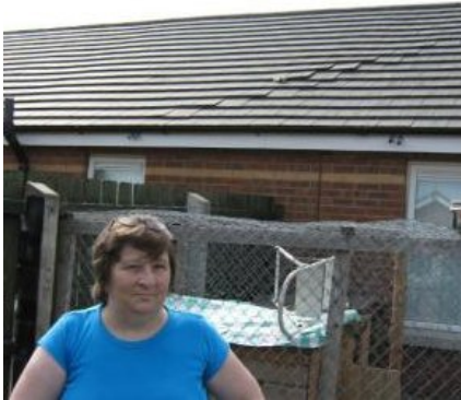
Belfast resident shocked by damage to tiles
